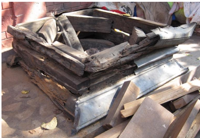
Fig 4 & 5: The extent of damage of the base structure of the Gajur and the Gajur (right).
